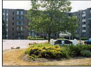
HIGHLAND WOODS HUD 223(f)/TPA 661 Suites Warrensville Heights, OH
